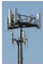
Wireless Base Station
