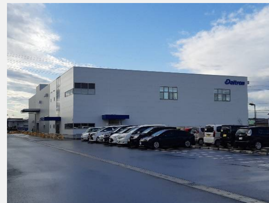
Photo of completed Chubu Second Factory
