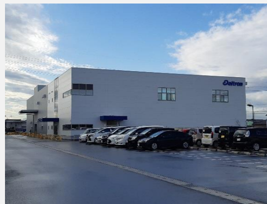
Photo of completed Chubu Second Factory
