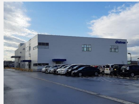
Photo of completed Chubu Second Factory
